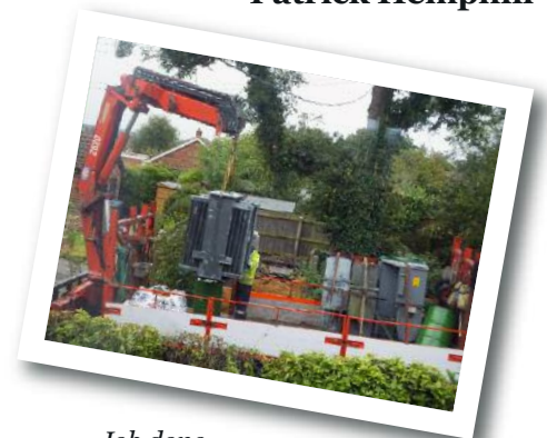
Job done. Removal of the old transformer
