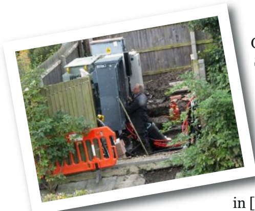
The new transformer being connected
